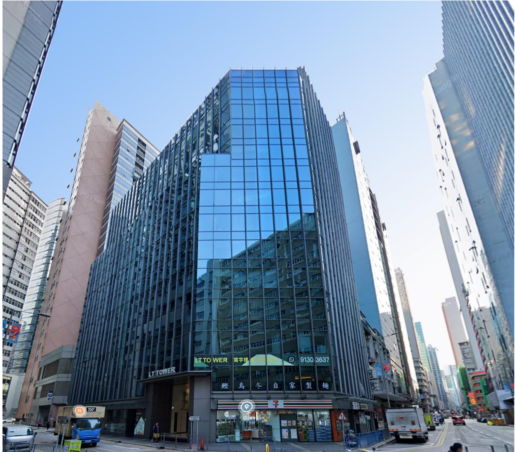
PHOTO 1 - Western facade of the building
